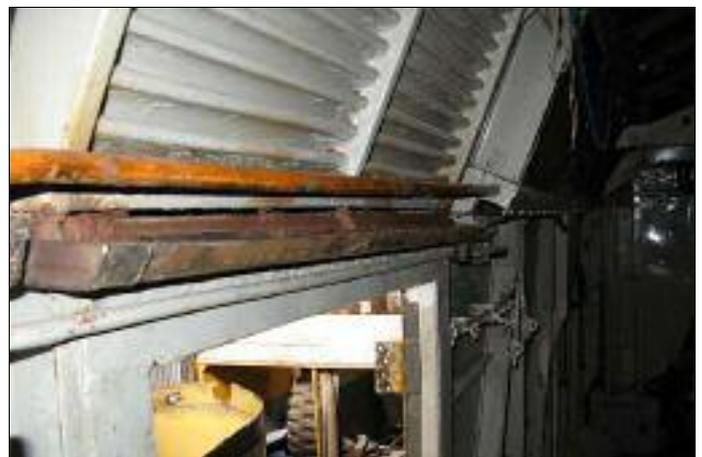
New internal gutters welded in place.
